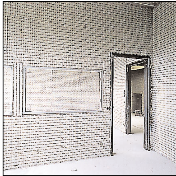
Walls in Stucanet® Poutrafil®, hospital St.-Jan (Bruges).
