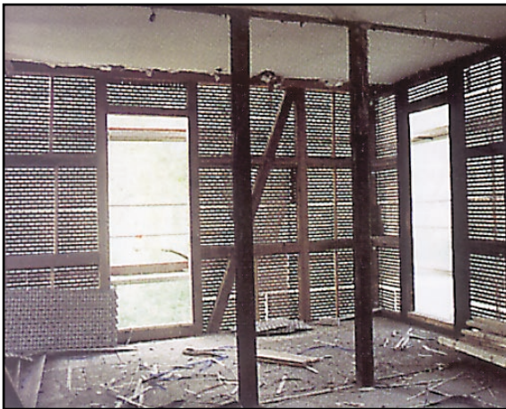
Tember frame construction, Germany.
