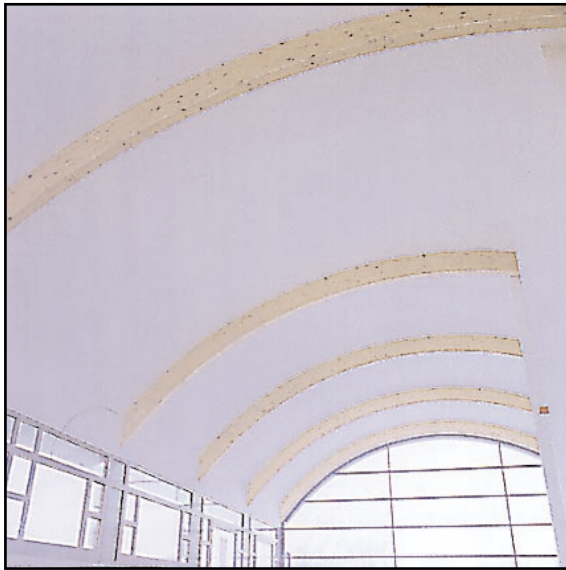
Bended ceiling construction - Shopping center, Brugge (Belgium).
