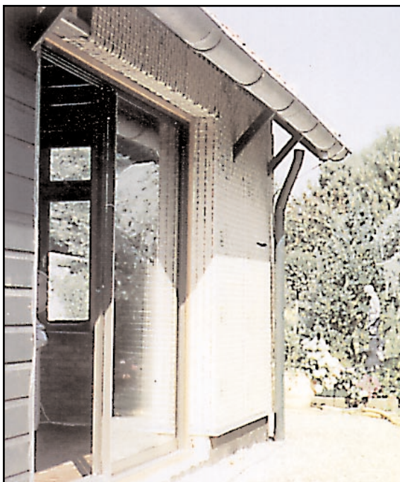
Renovation outer wall of a house in Vledderveen, Drenthe (Neth.).
