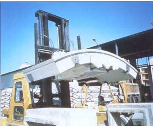
Transportation of precast segments (Metrosud).
