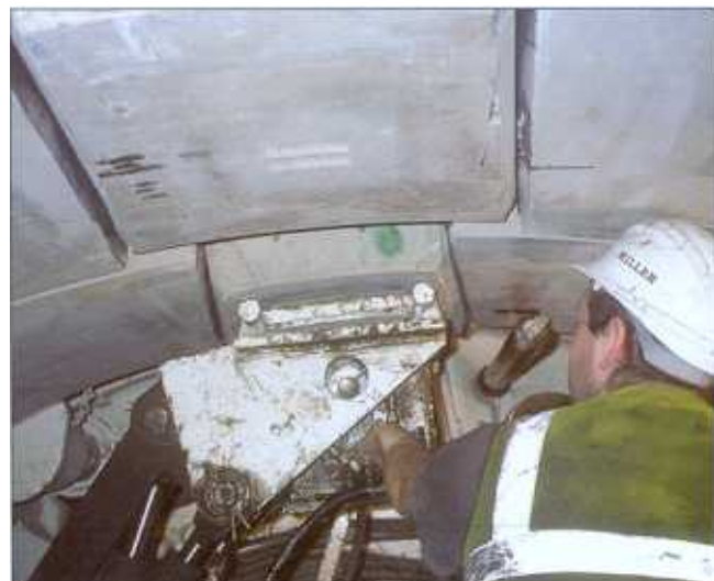
Installation of the key-segment (Heathrow).
