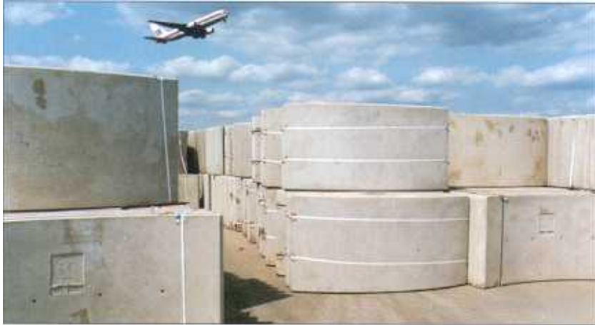
Vertical storage of segments (Heathrow).
