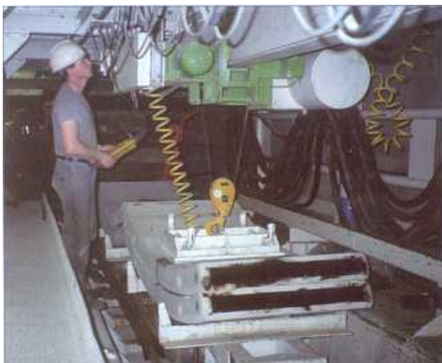
Handling of a segment (Heathrow).
