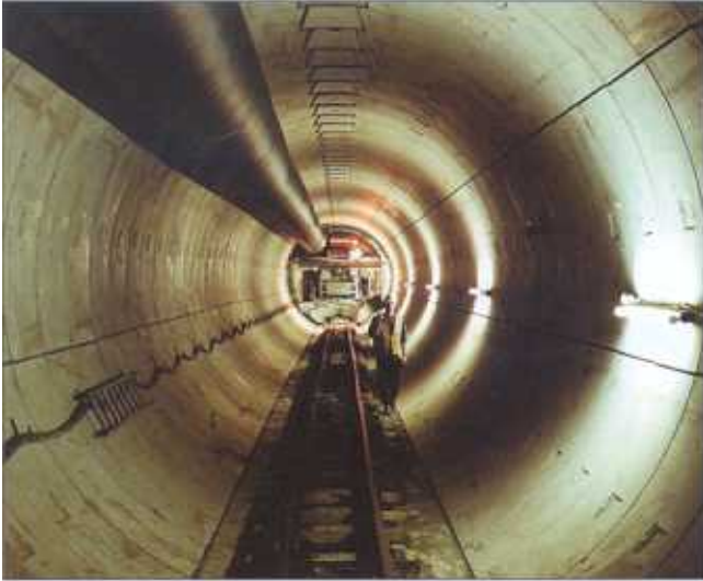
Baggage tunnel at Heathrow airport London constructed with Dramix® steel wire fibre reinforced concrete segments.
