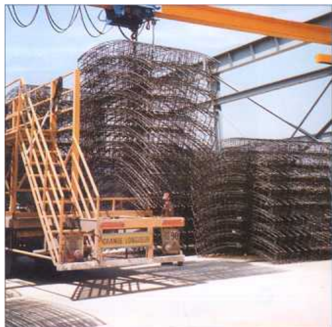
Unloading and stacking of reinforcement cages.
