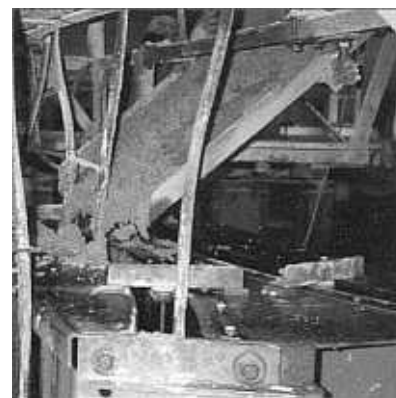
Pouring of the steel wire fibre reinforced concrete into the mould.
