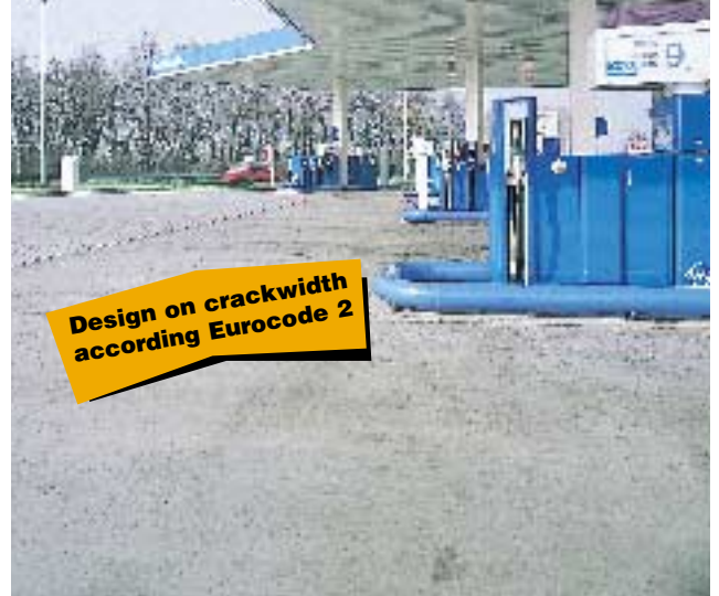
Petrol station according to most severe German guidelines (DAfStb-Richtlinie) with a fluid tight floor.
