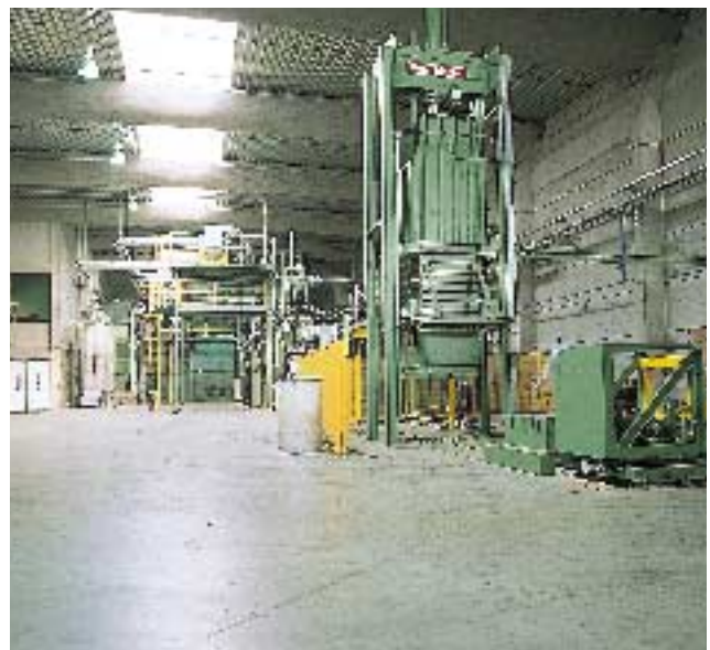
This production area needed a foundation for heavy machinery.
