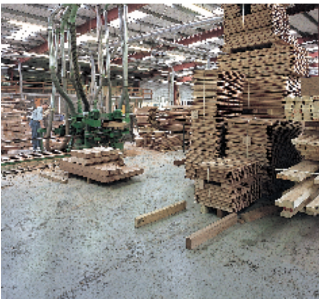
Workshop with high impact resistance and full flexibility for moving machinery around.
