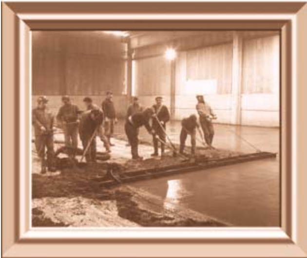
1976. Back to the past ... Labour intensive placing techniques of 20 years ago in a Bekaert production plant using Dramix® reinforcement.
